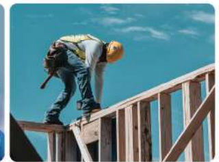
Factory & Construction site
