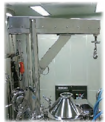
Cleanroom Jib Crane
