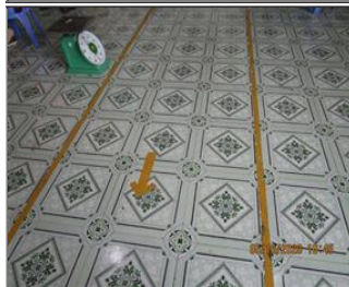
Photo of fire safety equipment Exit route.JPG
