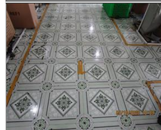
Photo of fire safety equipment Exit route.JPG
