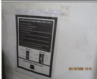
Photo of fire safety equipment Instruction of using fire extinguisher.JPG
